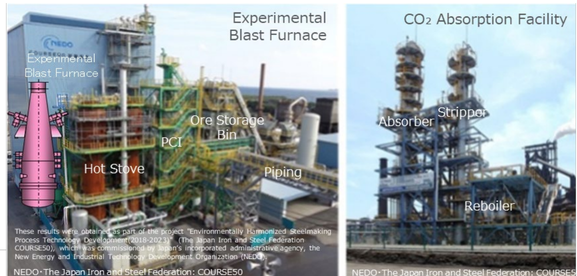
Experimental Blast Furnace and CO 2 Absorption Facility (COURSE50)
